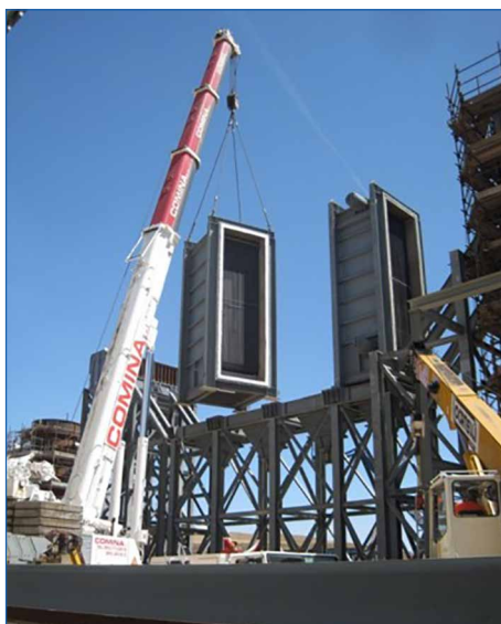
Figure 9: Typical modular boiler assembly
