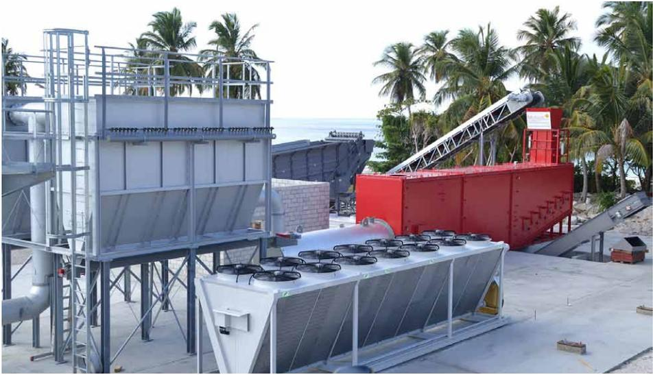
Figure 6: View to the incinerator, back house filter and air cooler
