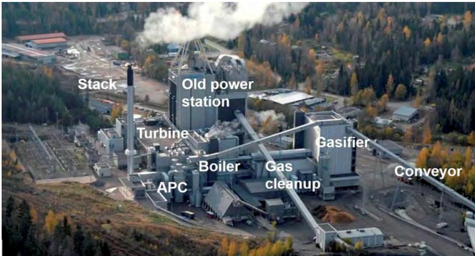
Figure 4: Lahti gasification power plant
